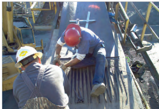
Conveyor belt maintenance
